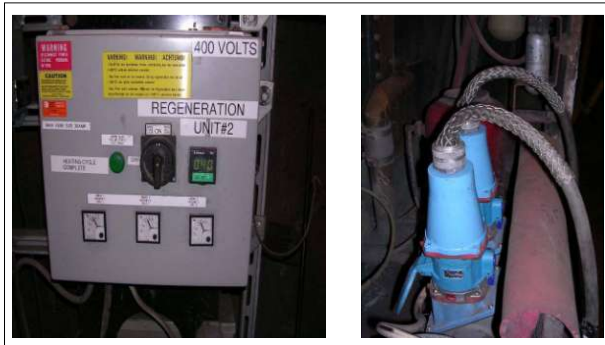
Figure 46: Regeneration control panel for one of the ECS Combifilters (left) and power cables connectors (right).
