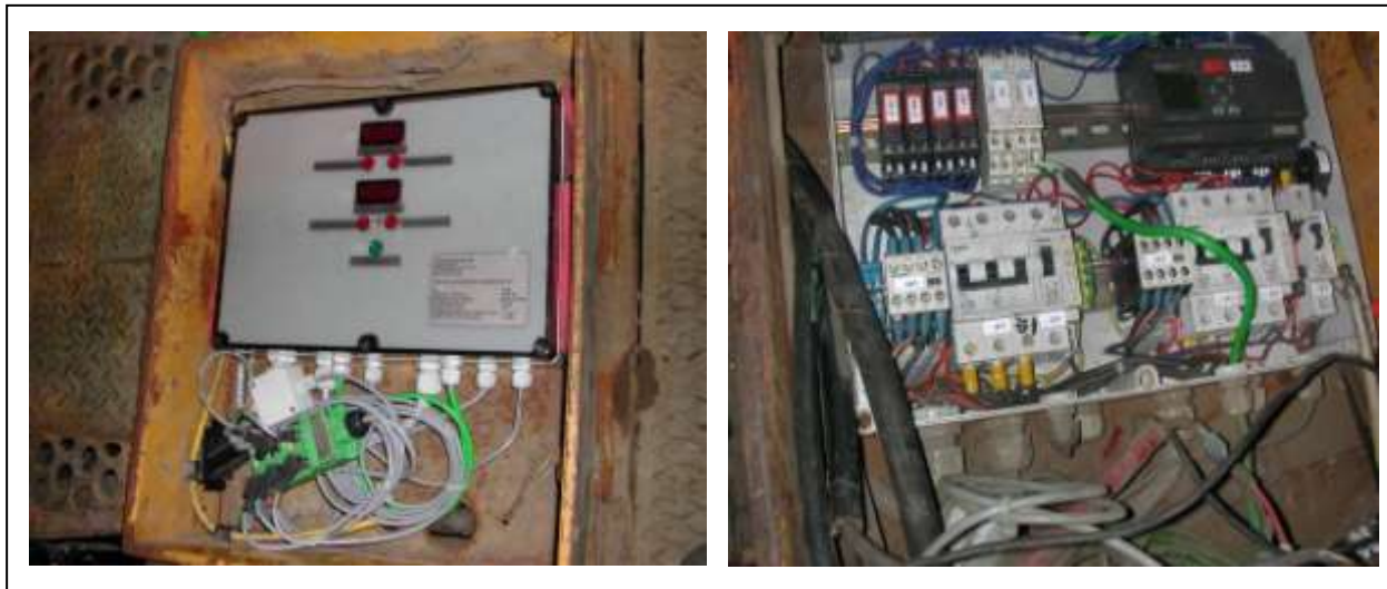
Figure 30: JM electric regeneration control display panel (on left) and interior (on right).
