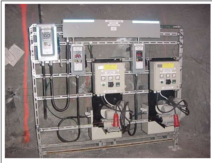
Figure 45: Regeneration control station for the DPF system using dual ECS Combifilters.
