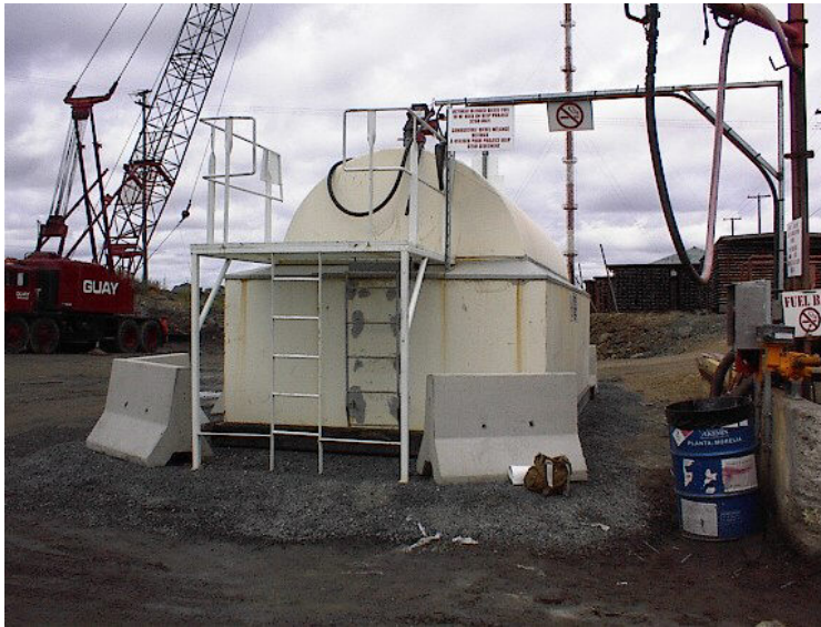
Figure 21 - Blended Fuel Storage on Surface
