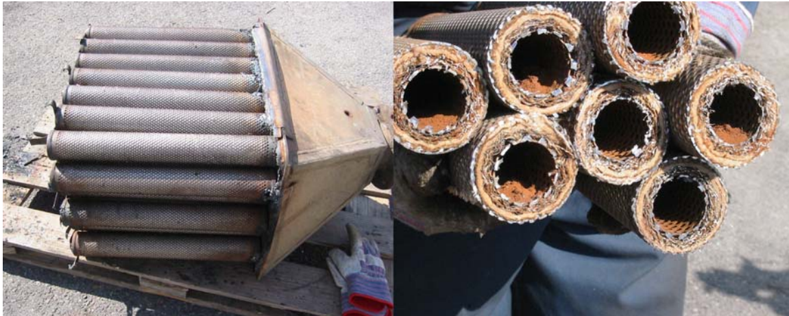
Figure 54 - Oberland Mangold Fiber Cartridges and Iron Oxide Accumulation
