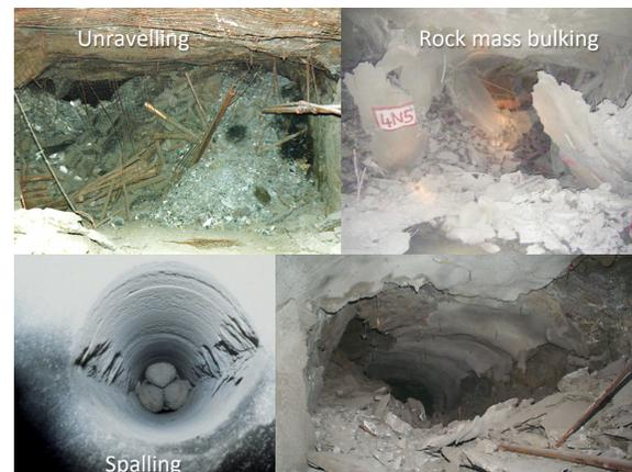
Figure 2 Examples of excavation instabilities in stressed rock.
